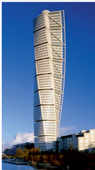
Turning Torso Malmö/Sweden
